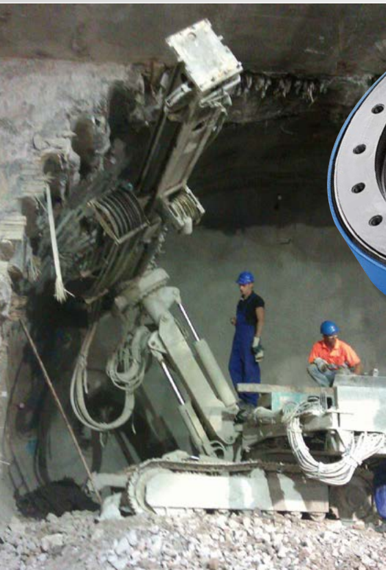
Slew drive in the WD-L range for a special device for insertion of wall reinforcement
